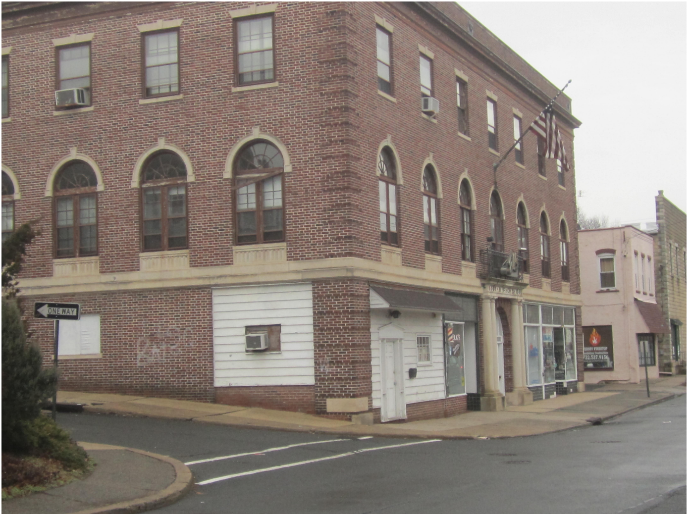
Corner view of 305 East Second Street
