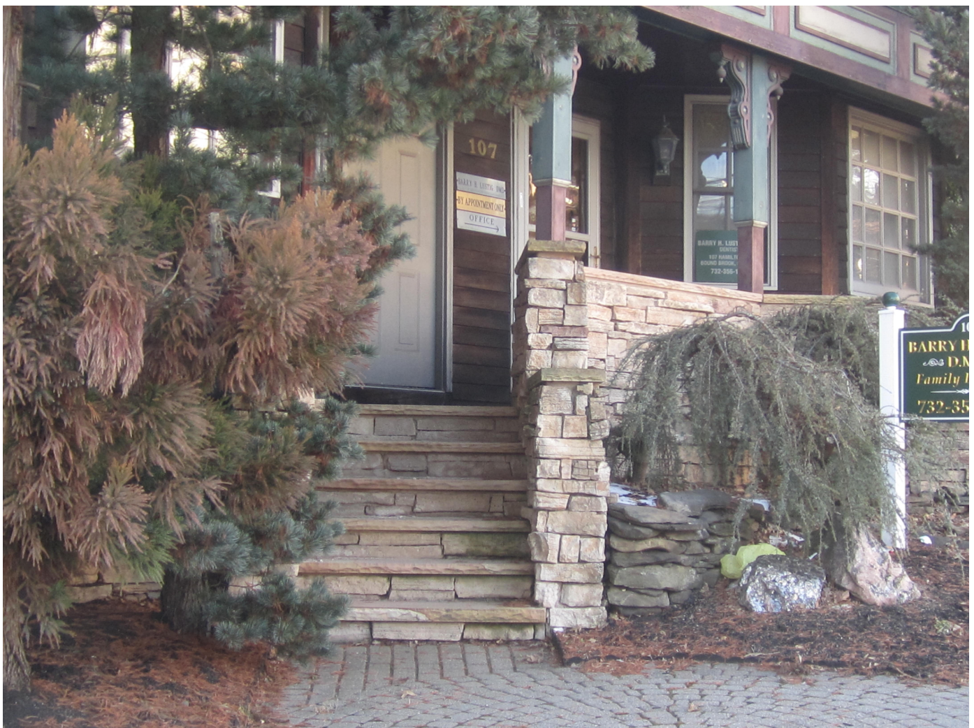
Front view of 107 Hamilton Street
