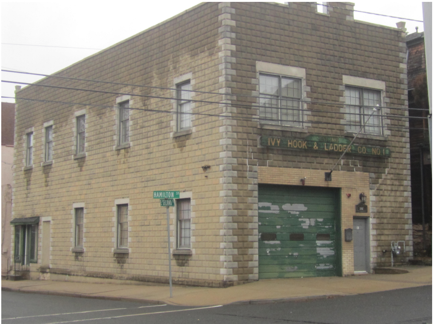
Angled view of 103 Hamilton Street
