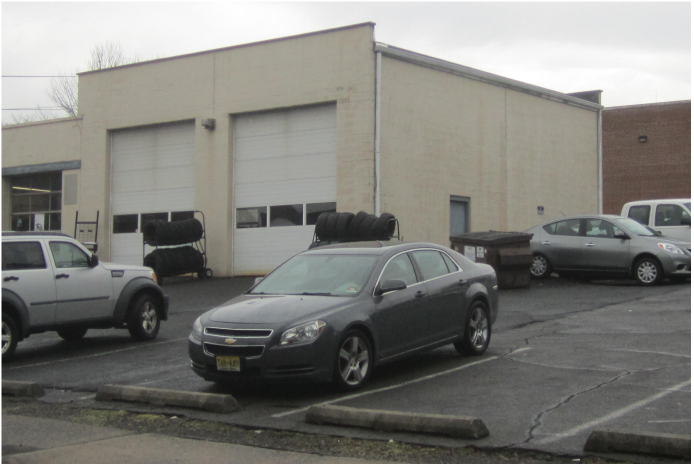
Side view of 203-209 East Second Street
