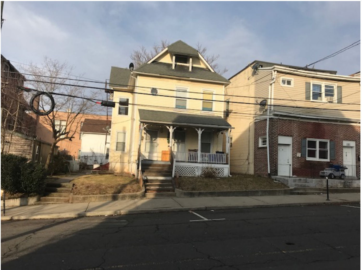
Front View of 109 Hamilton Street.
