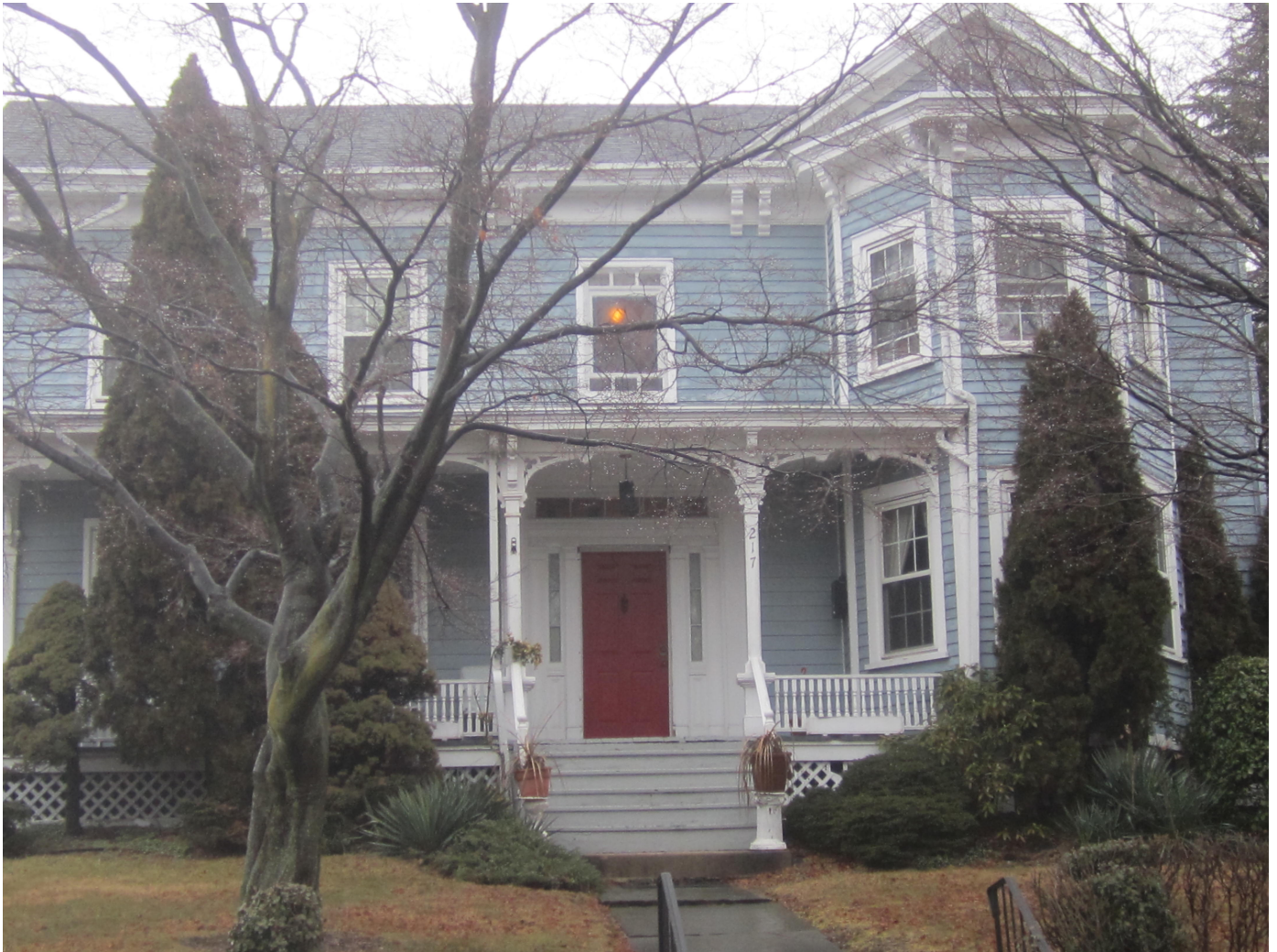
View of front of 217 East Second Street
