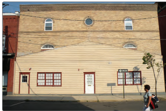
Inappropriate building alterations should be removed, where possible, and the original building facades restored.
