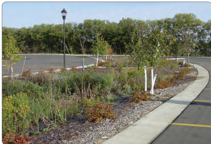
Rain gardens and permeable pavements soften the built environment and perform valuable water quality and recharge functions.
