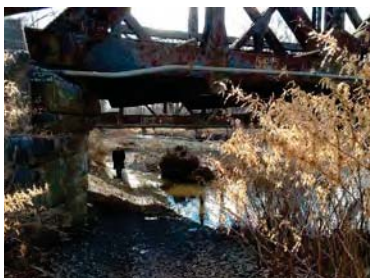
Fig 40. Path Under Trestles
