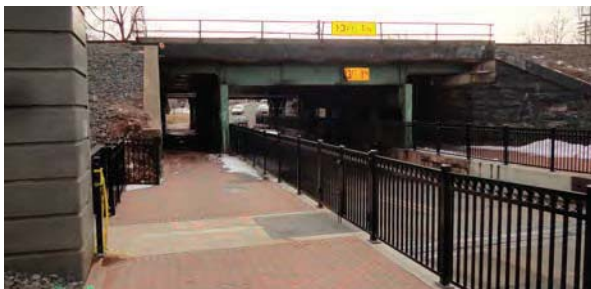
Approach to pedestrian underpass
