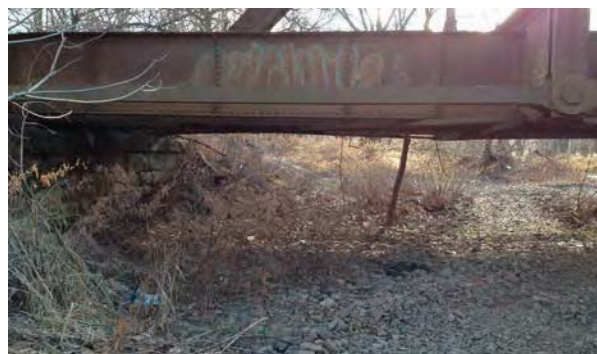
Limited clearance under Middle Brook Crossing
