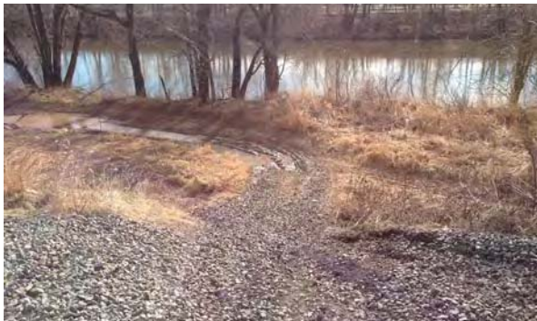
(1) Some trail users climb this embankment to the active rail ROW
