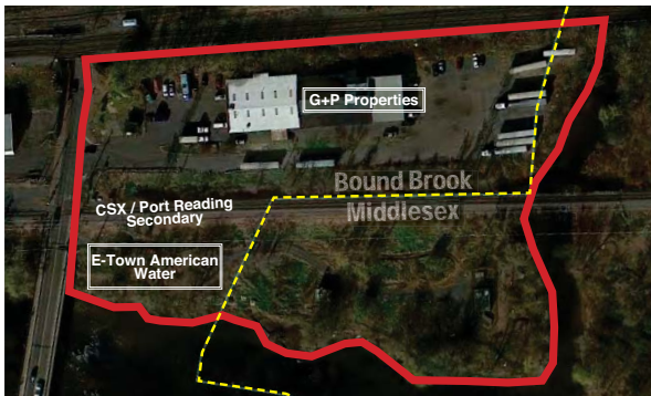
Existing Conditions Aerial Photograph
