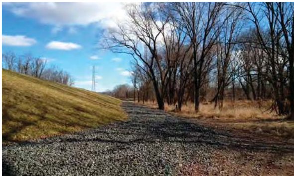
Gravel path at base of levee (looking SE)
