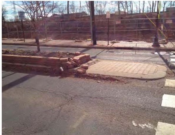
Roundabout: Median in disrepair.
