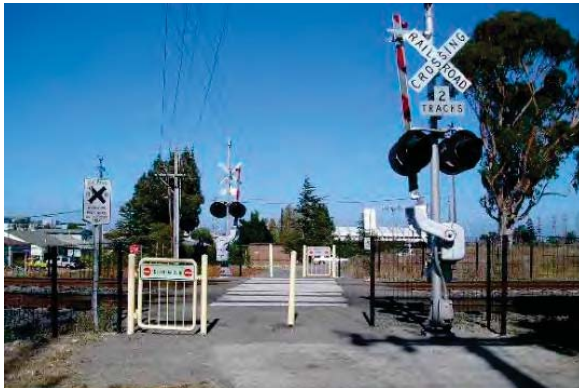
Fig 34. Pedestrian Crossing with Safety Lights And Gates
