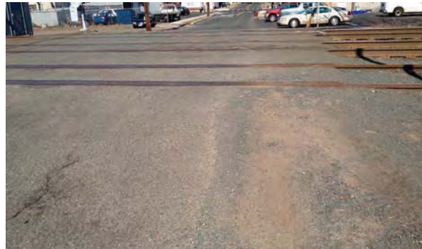
Vosseller Avenue rough asphalt surface between rails
