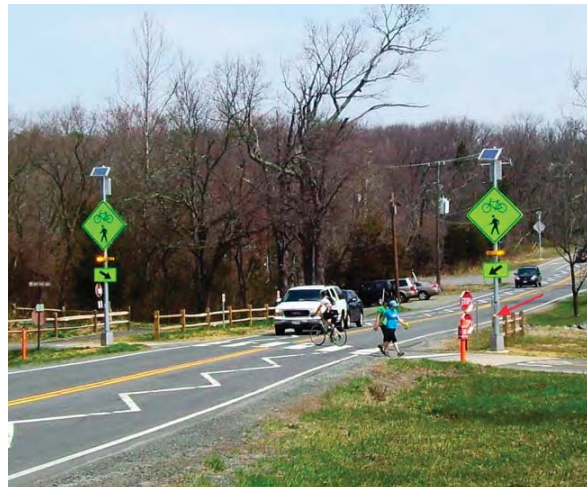
Fig 11. Rectangular Rapid Flashing Beacons at Trail Crossing
