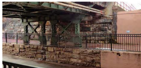
Interesting stone walls and steel trusses
