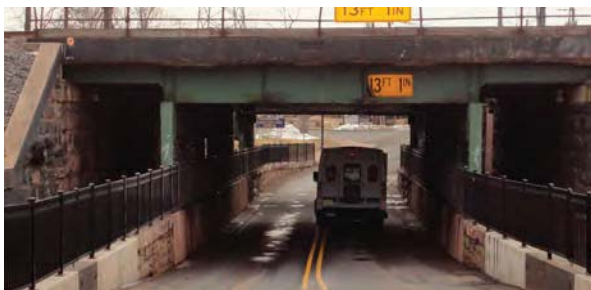
Vehicles are grade separated from pedestrians
