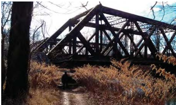
Trail beneath Middle Brook rail road bridge
