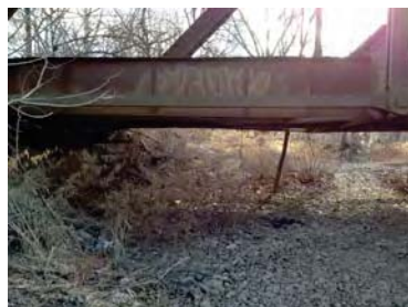
Fig 41. Limited Head Clearance
