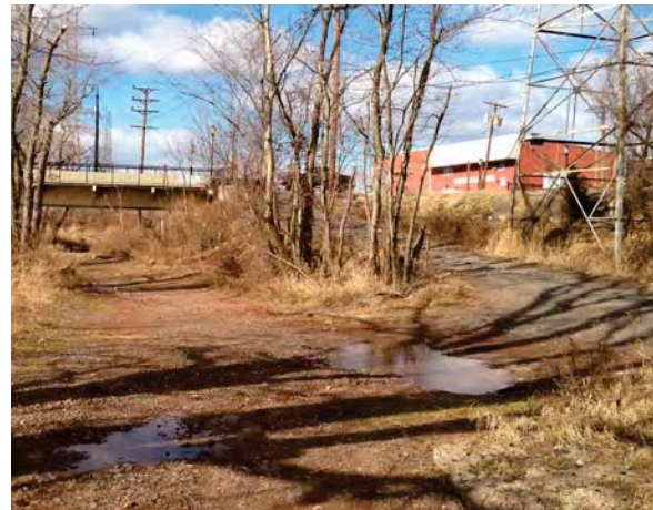
View looking west under Queens Bridge with Conrail access drive on right
