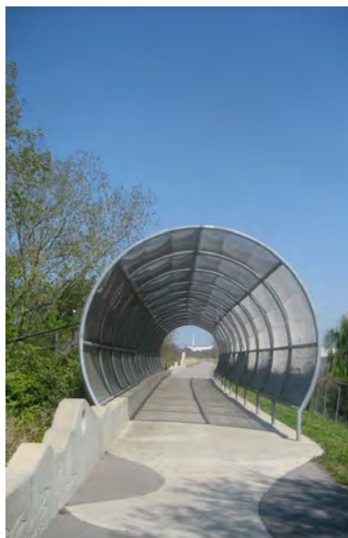
Shade Screen Tunnel
