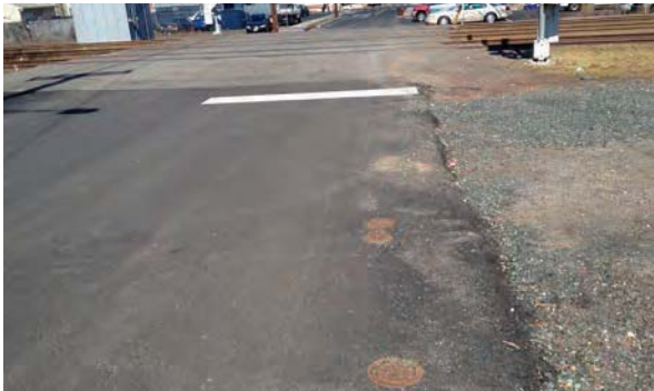
Vosseller Avenue edge condition and lack of sidewalks.
