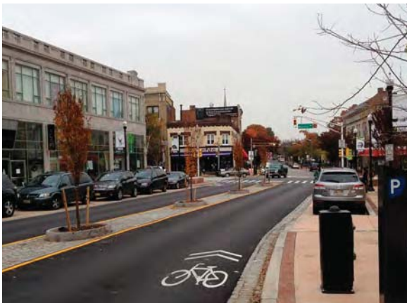
Share the road painted symbols (Sharrows) as well as signage will make drivers aware the bicyclists will be using this road (Montclair, NJ).
