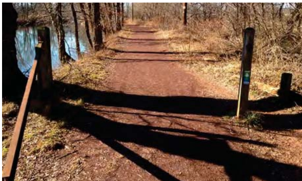
Crushed Stone Trail
