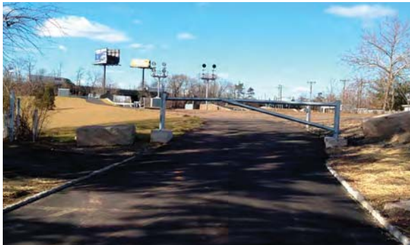
Gate at W. Main Street access to maintenance path
