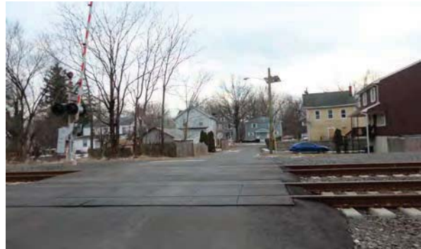
Lamonte Avenue new crossing surface
